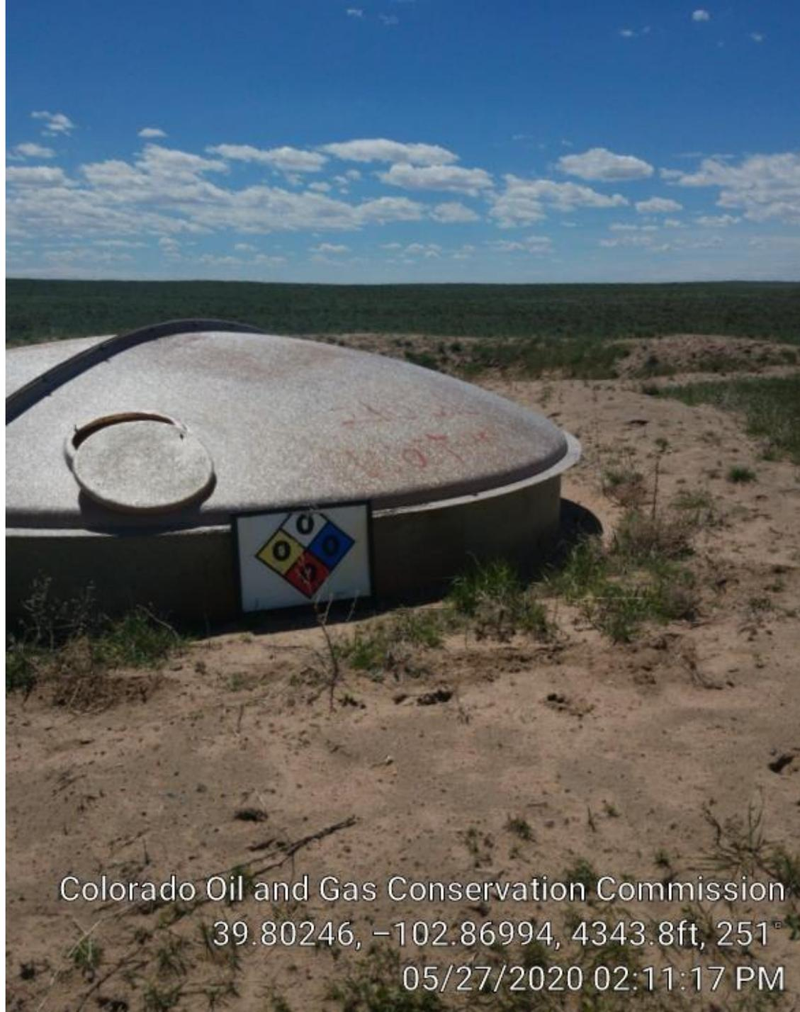
Bird cover needs to be completely closed, NFPA sign for produced water has to have at least 1 for dissolved gas, and maintain tank labels for quantity and contents.
