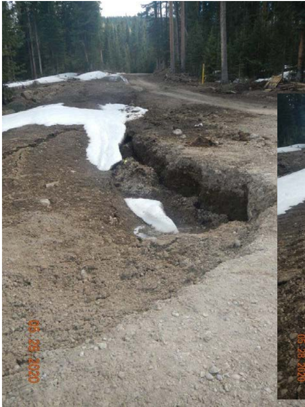
Photo#6: Cracking /sloughing at entry.
