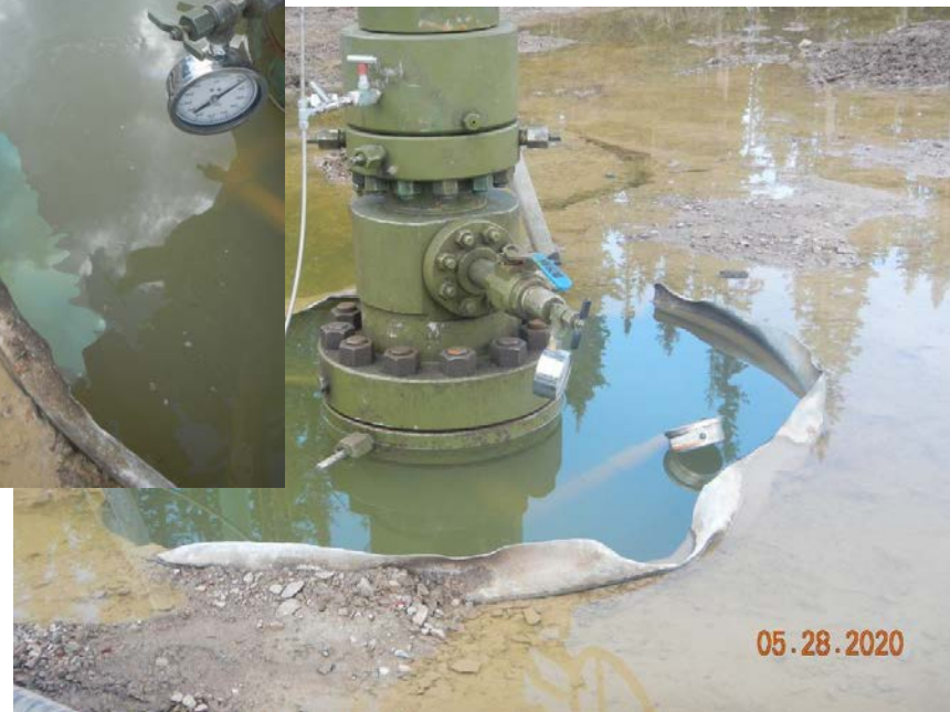
Photo#11: Cellars over flowing with stormwater.
