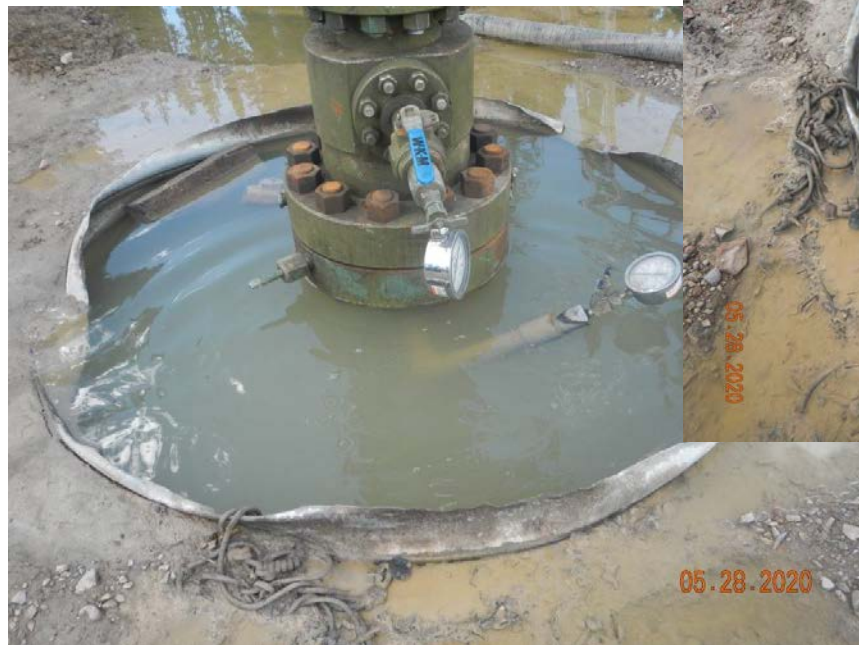
Photo#10: Cellars over flowing with stormwater.
