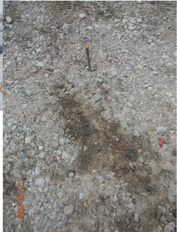
Photo#17: One of several rebar protruding from pad surface
