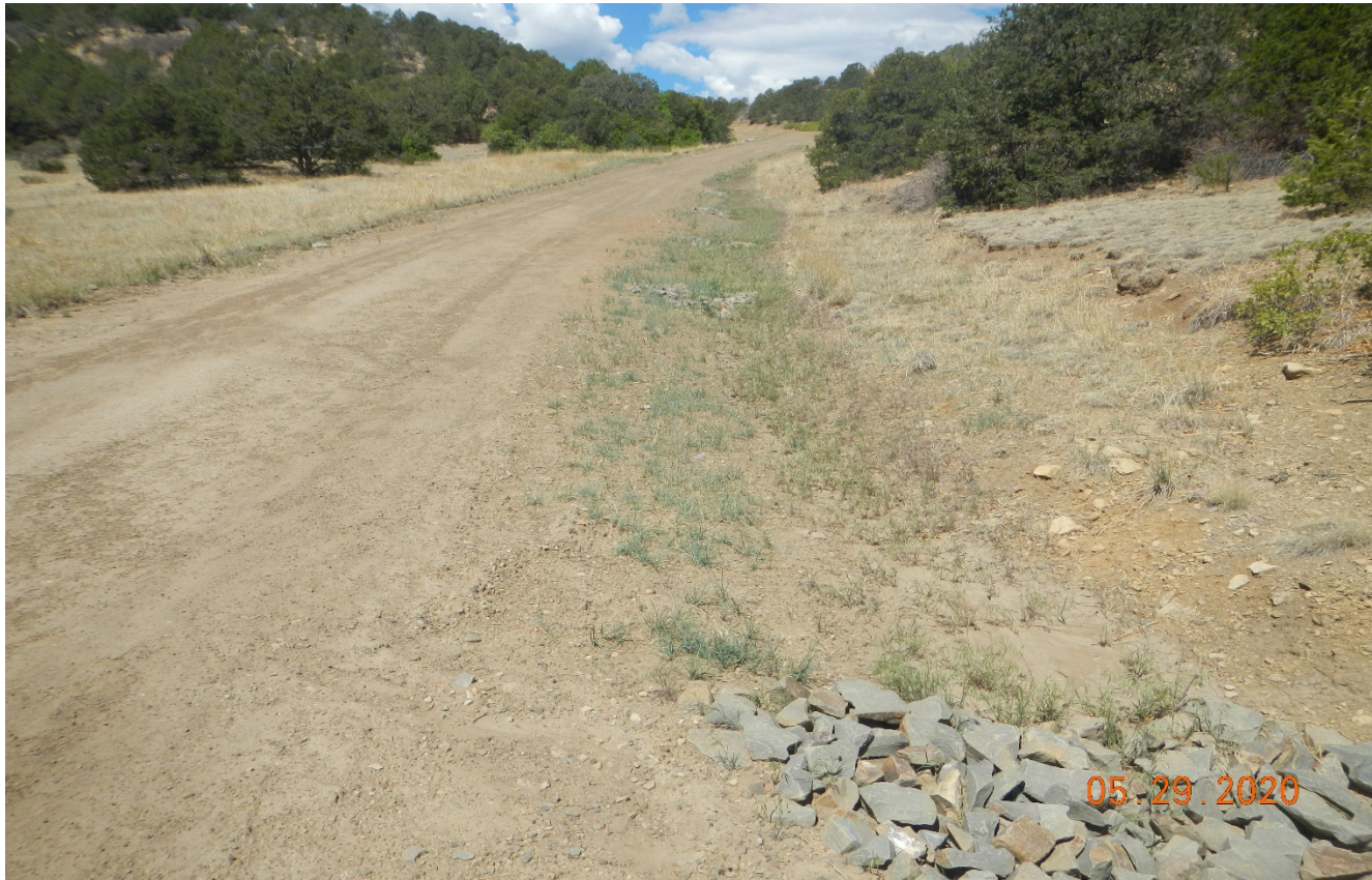
Photo 1. Facing west along the main road near the location. The road is stabilized and BMP's are installed along the road.
