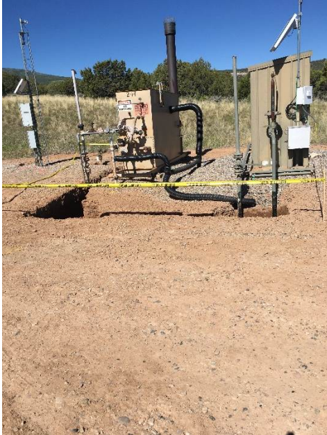
A new 2" Stainless steel flow line will be installed from separator to gas meter, Approximately 20'
