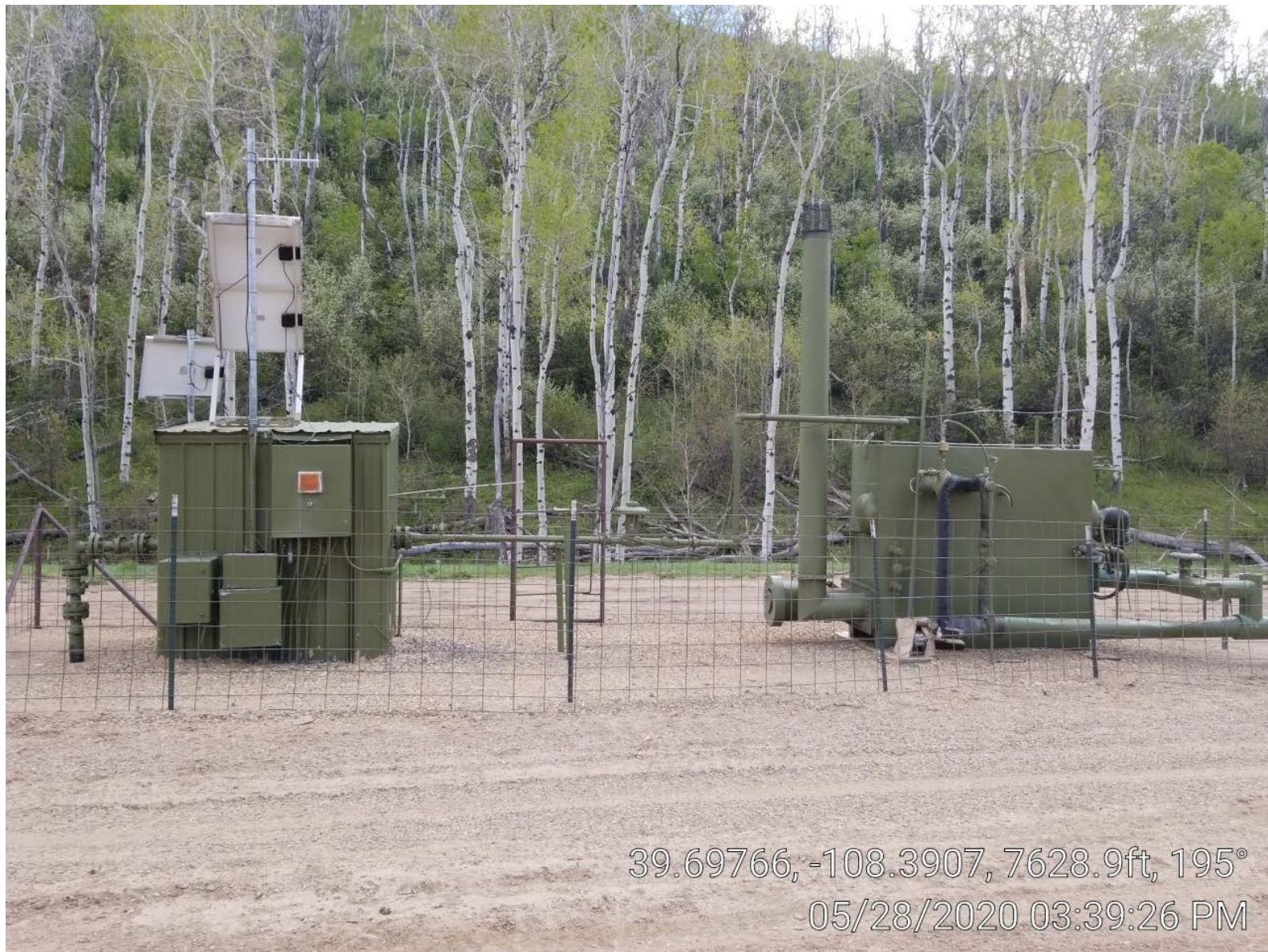
Photo 3. Separator & meter building.
