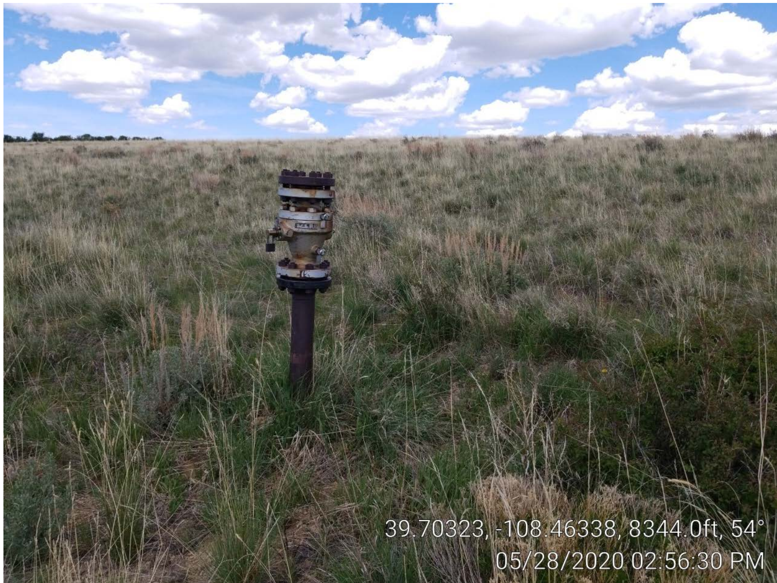
Photo 2. Flow line riser at edge of location.
