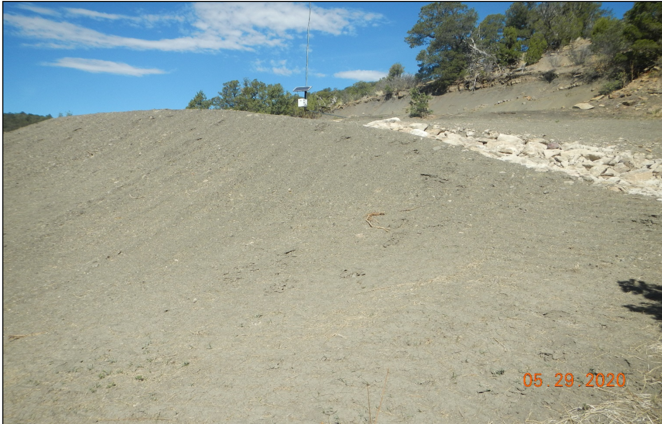
Photo 4. Facing northwest toward the pit. The disturbed soils have been seeded and temporarily stabilized by tracking.
