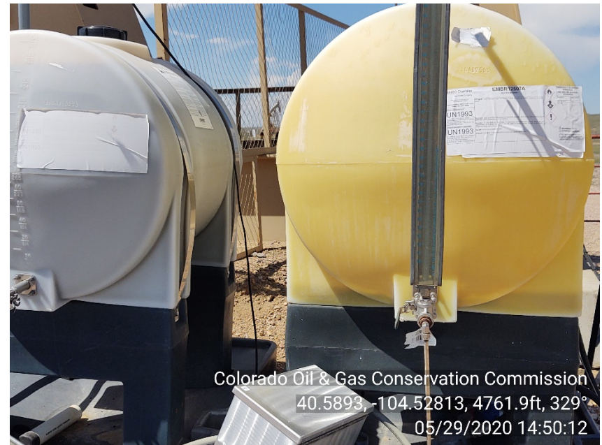
Photo #4 Dillard AB 10-08 Wellsite Faded Container labels Faintly legible : Consider replacing
