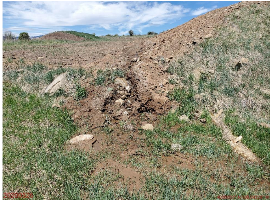
Photo 6: Photo taken from the southwest end of the Location, facing north. Photo shows area where perimeter stormwater diversion ditch discharges from the Location; BMP has not been constructed in accordance with good engineering practices, or with a sufficient stabilized outlet to prevent degradation, and allow for sediment laden-free stormwater discharge from the Location; Erosion degradation evident with off-site sediment transport and deposition occurring
