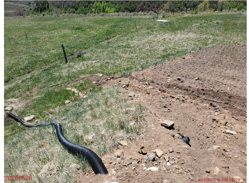
Photo 4: Photo taken from the southwest end of the Location, facing southwest. Photo shows area where perimeter stormwater diversion ditch discharges from the Location; BMP has not been constructed in accordance with good engineering practices, or with a sufficient stabilized outlet to prevent degradation, and allow for sediment laden-free stormwater discharge from the Location; Erosion degradation evident with off-site sediment transport and deposition occurring
