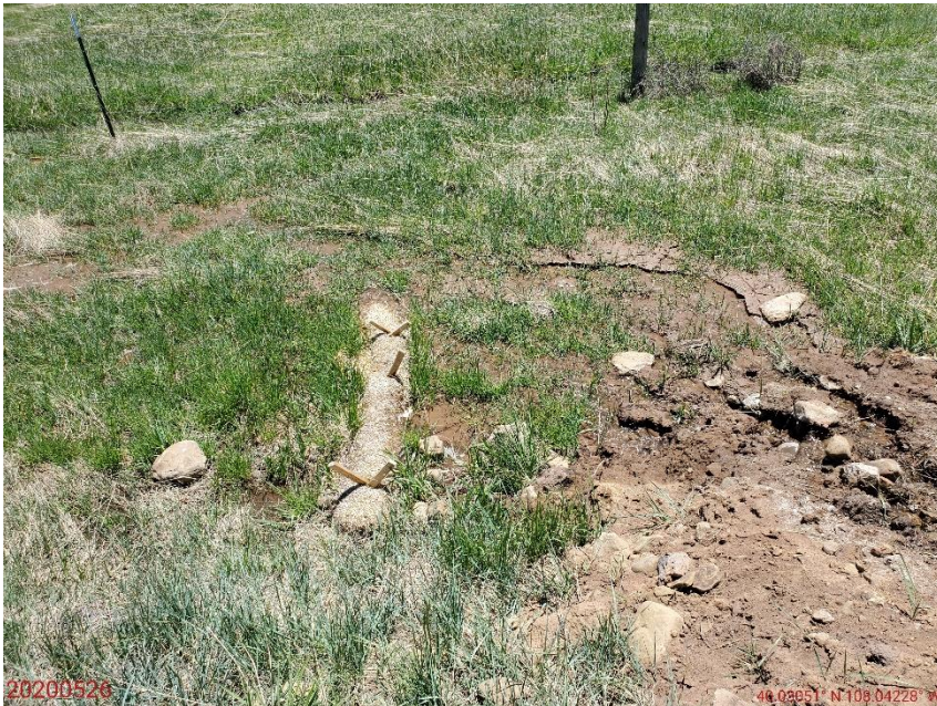
Photo 5: Photo taken from the southwest end of the Location, facing south. Photo shows stormwater erosion and off-site sediment transport and deposition occurring
