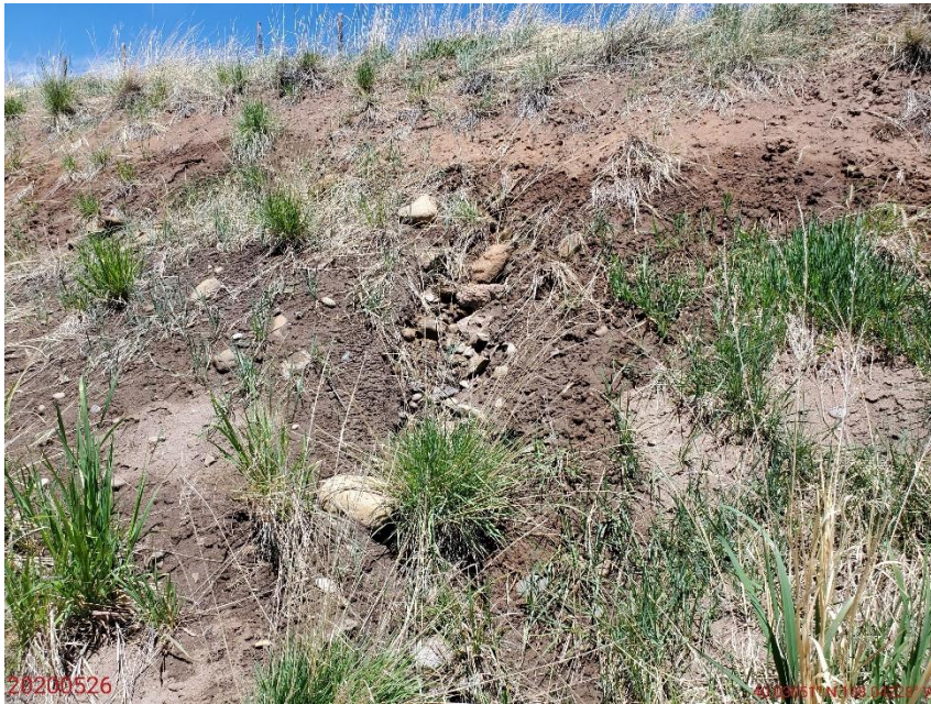
Photo 3: Photo taken from the cut slopes on the northern end of the Location. Photo shows a seep appears to have developed in the cut slope resulting in water discharging and erosion degradation.
