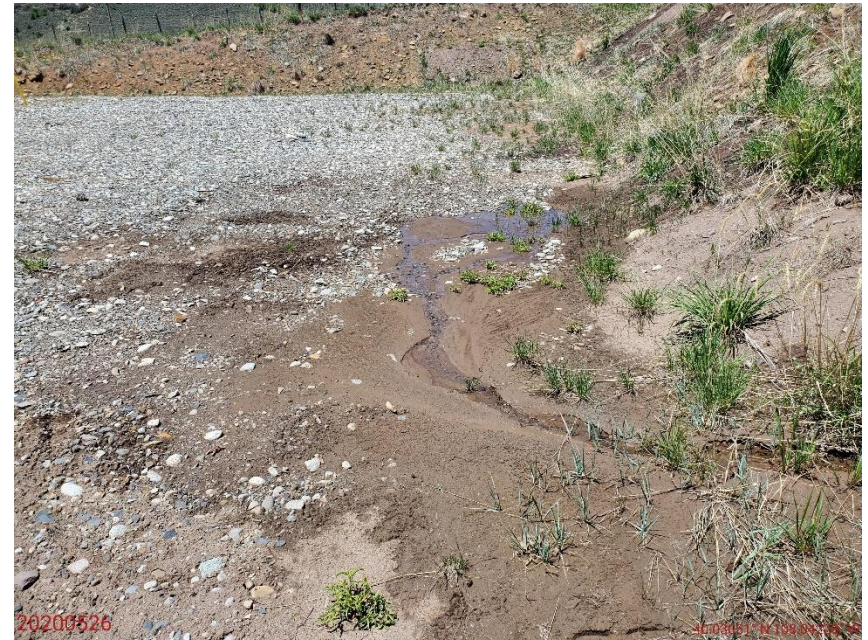
Photo 4: Continued from photo 3. Photo shows erosion degradation/sediment deposition on the pad from the cut slope
