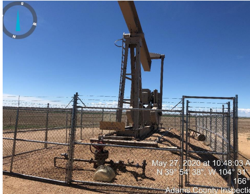
Photo #3 Pump Jack
