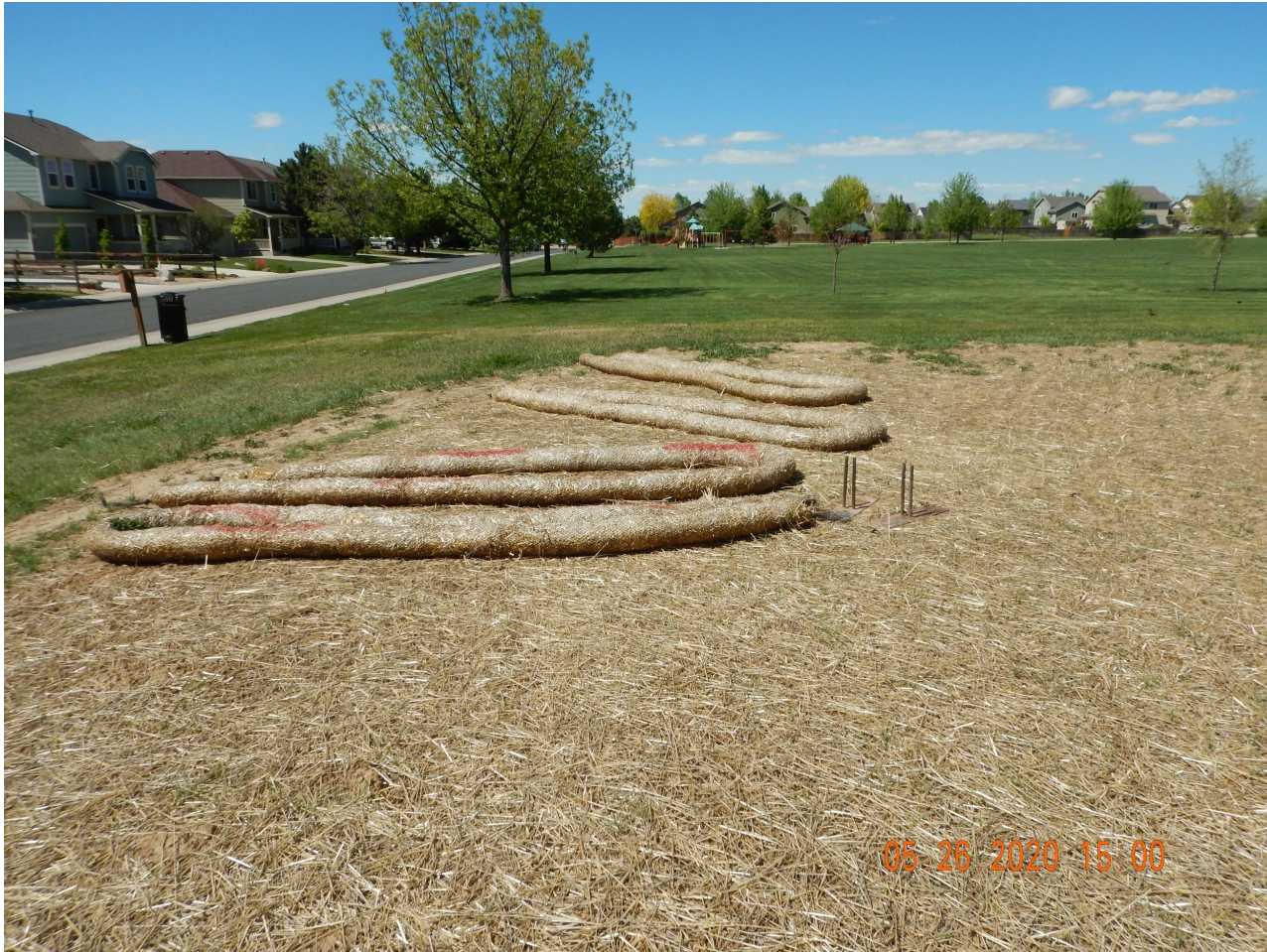
Photo 5. Photo taken from the northwestern location, facing North. Photo illustrates stormwater BMPs that appear to be decommissioned. Operator shall remove all unused materials if no longer needed.
