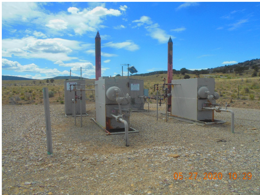
Separators and Meter housings
