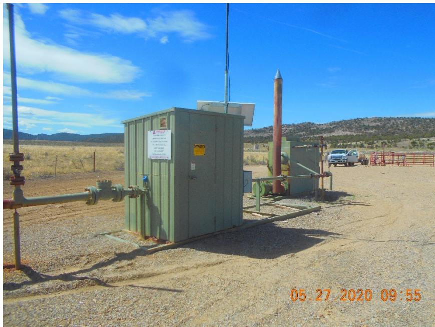
Meter housing with sign and separator
