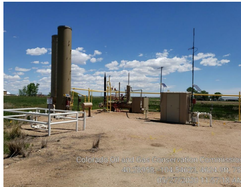
Photo #3 Separator, ECD's & Meter Run
