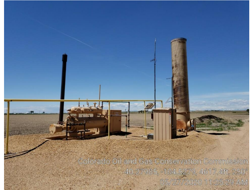
Photo #2 Separator, ECD & Meter Run
