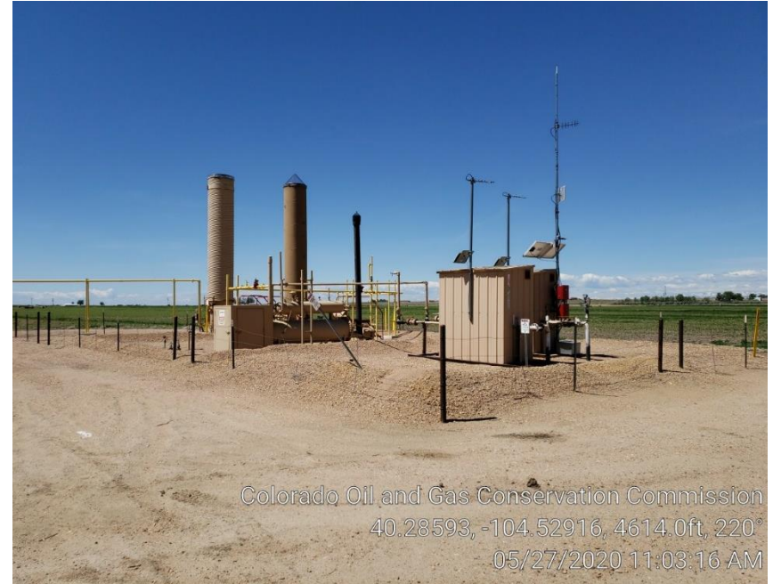
Photo #2 Separator, ECD's & Meter Runs
