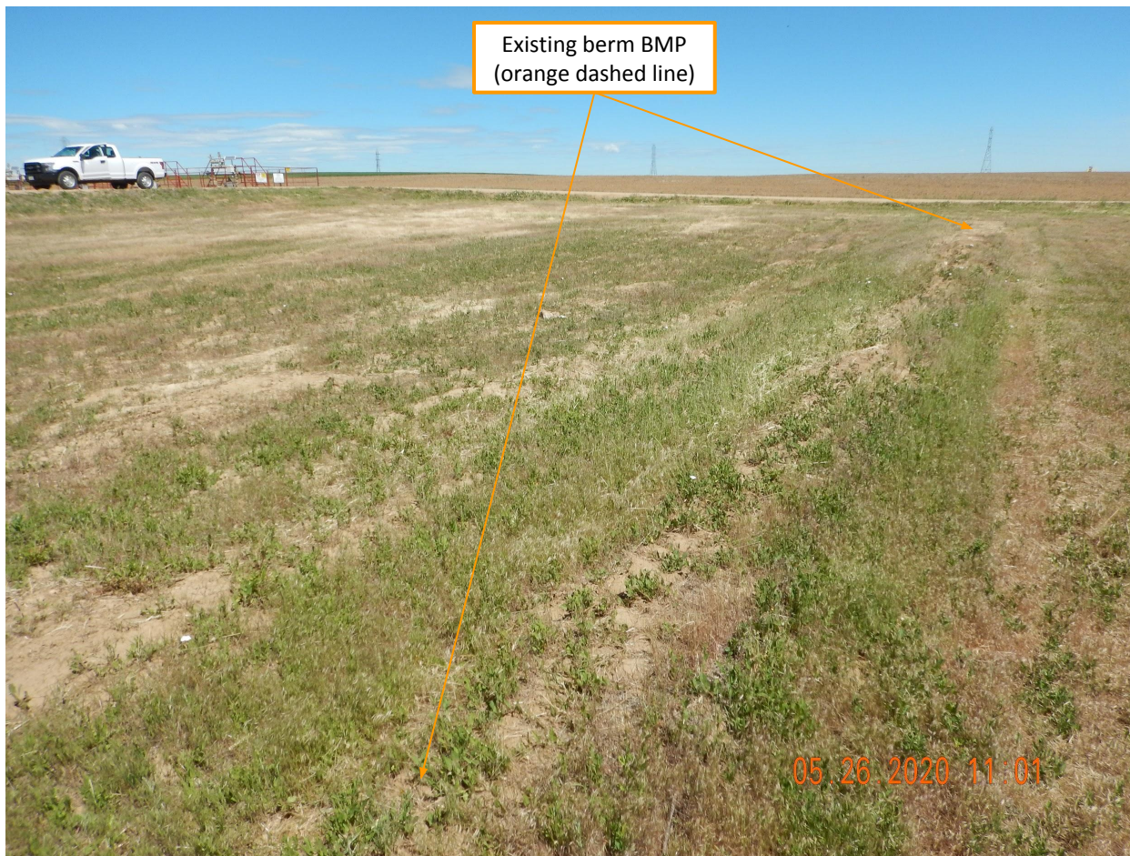
Photo 6. Photo taken from the eastern interim reclamation area, facing North. Photo illustrates a berm BMP that remains from construction operations along the eastern perimeter of the interim reclamation area. Sediment discharge has not gone beyond the berm BMP.
