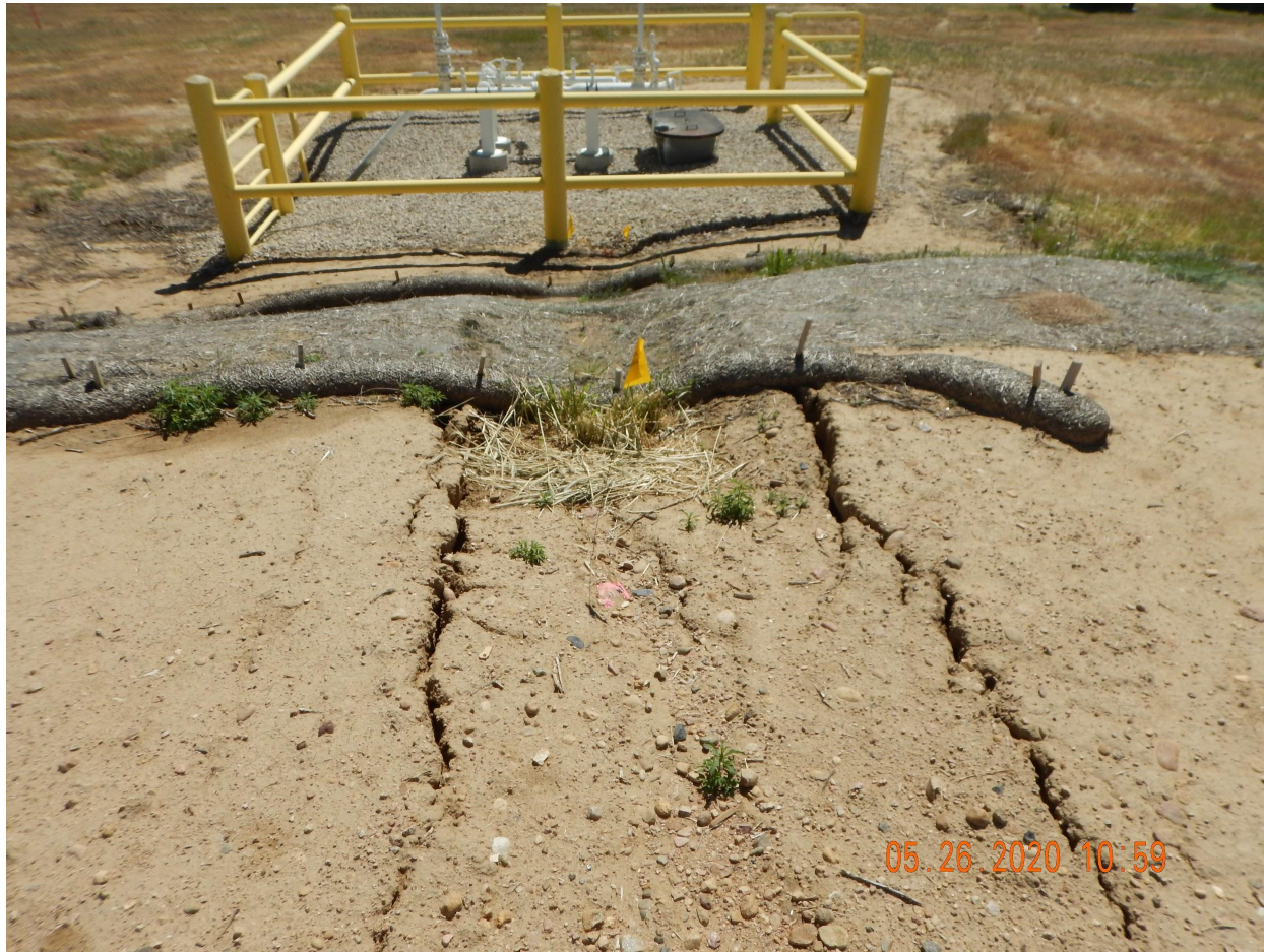
Photo 5. Photo taken from the southeastern location, facing East. Photo illustrates erosion and stormwater BMP maintenance required.
