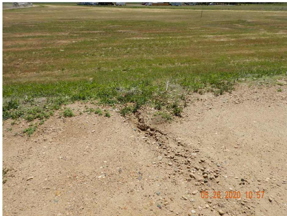
Photo 3. Photo taken from the eastern location, facing East. Photo illustrates rill erosion along the eastern fill slope. More erosion off other portions of the eastern location were observed.
