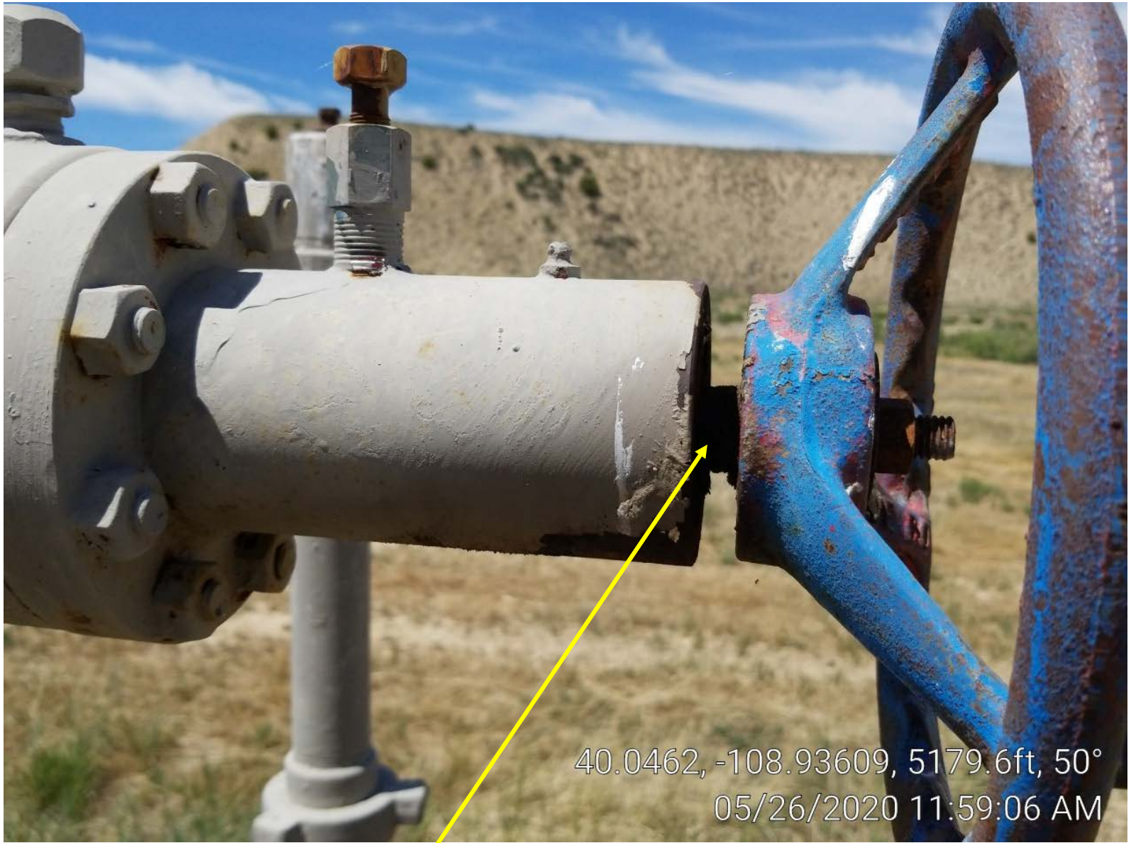
Photo 6. Casing valve gas leak.
