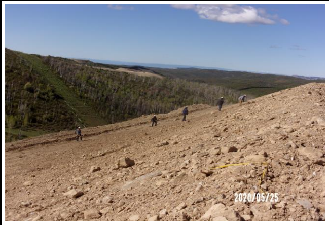
Erosion Repair on the C.C.604-12-13 Annex Pad
