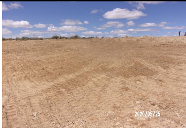
Erosion Repair on the C.C.604-12-13 Annex Pad
