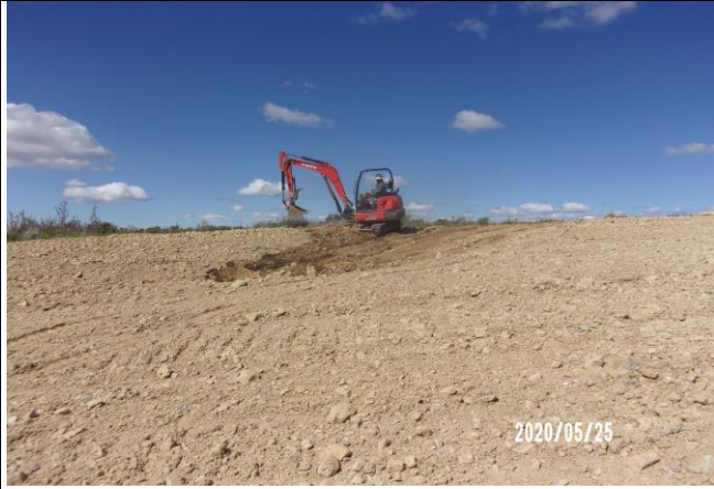
Crack Repair on the C.C. 604-12-13 Annex Pad
