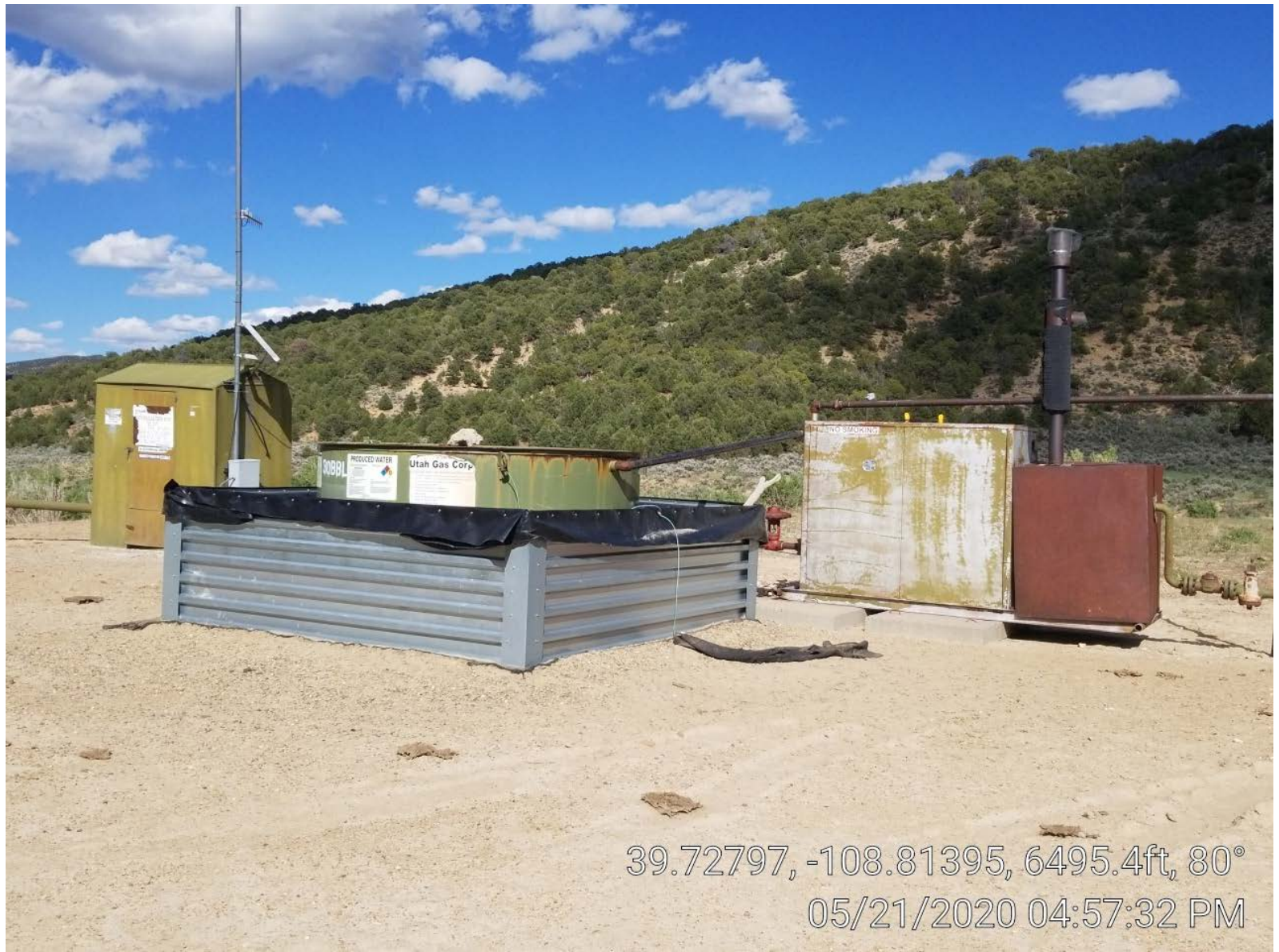
Photo 3. Meter building, tank, separator.
