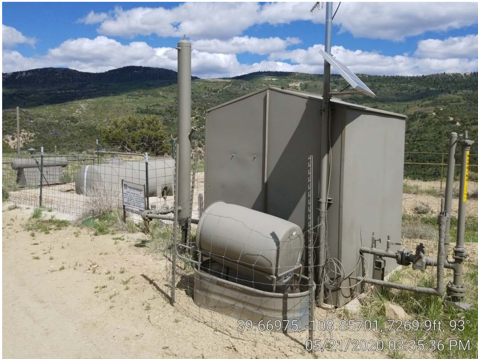
Photo 3. Meter building, tank, separator.
