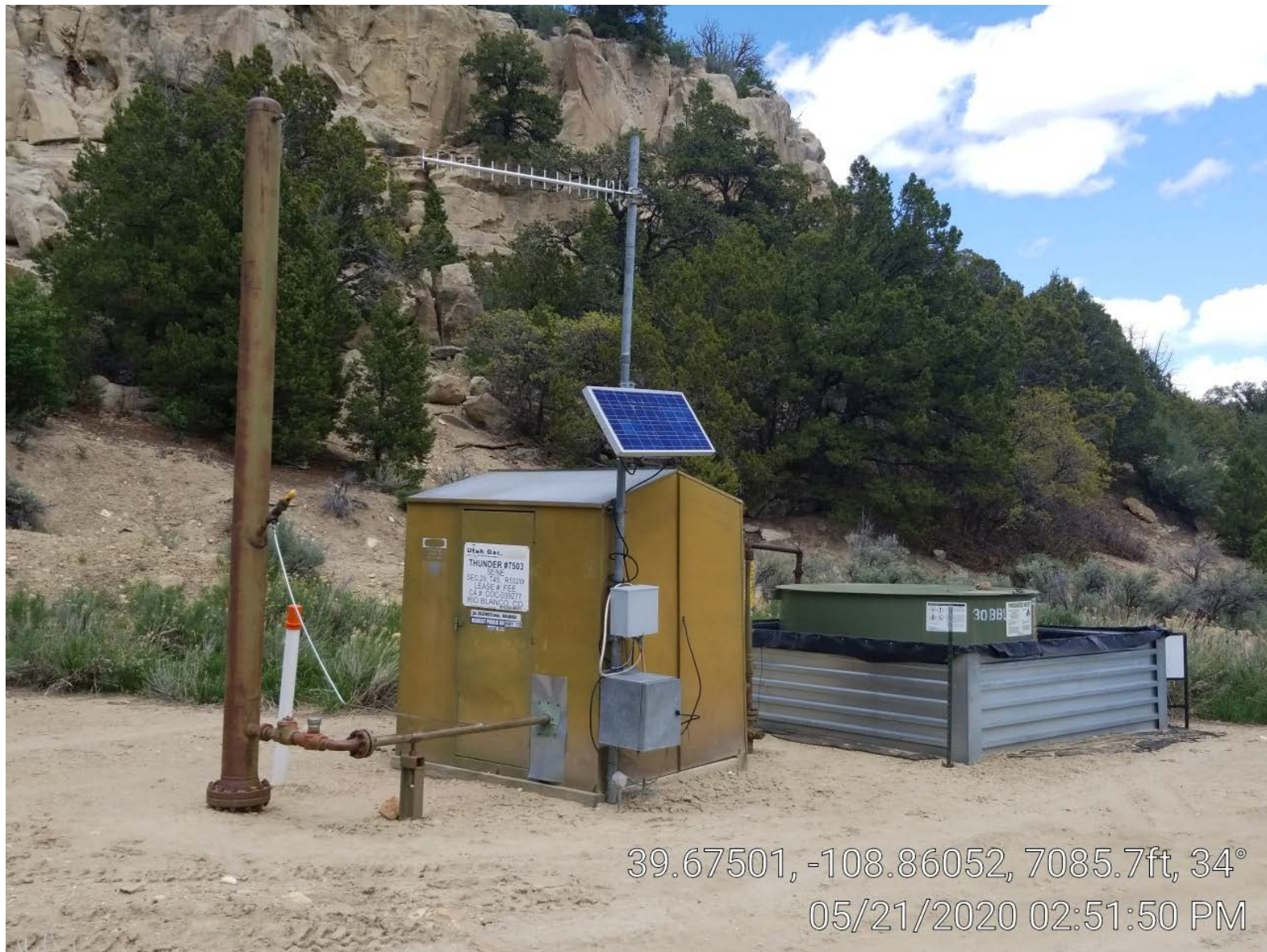
Photo 3. Separator & tank.
