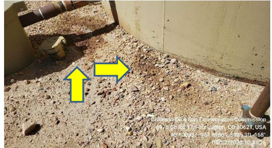
Photo 11 stained soil under split load out valve
