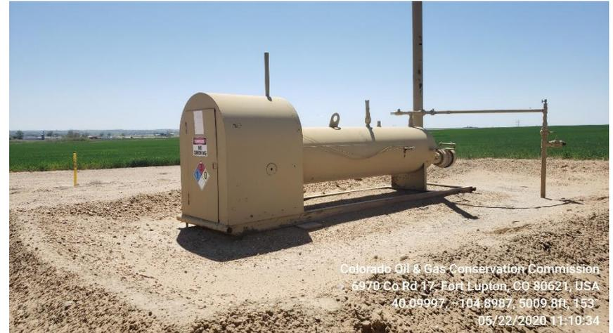
**Photo 7 Flow line manifold**
