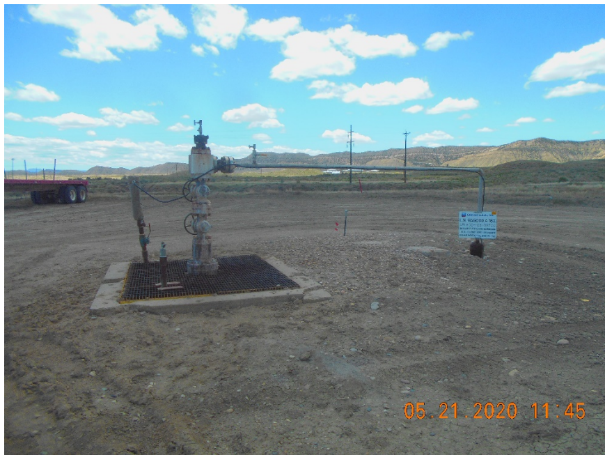
Injection wellhead
