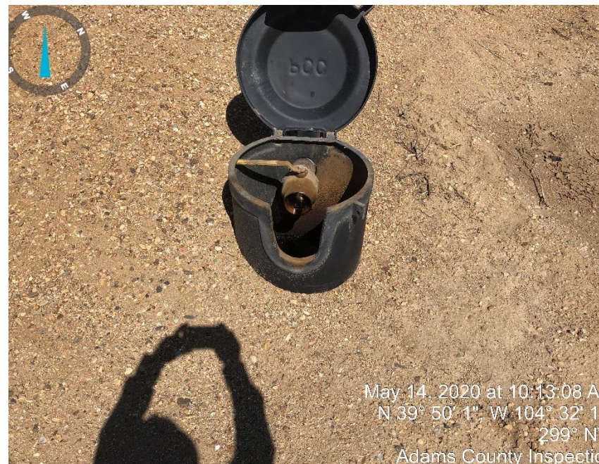
Photo #8 Bull Plug missing from load out line
