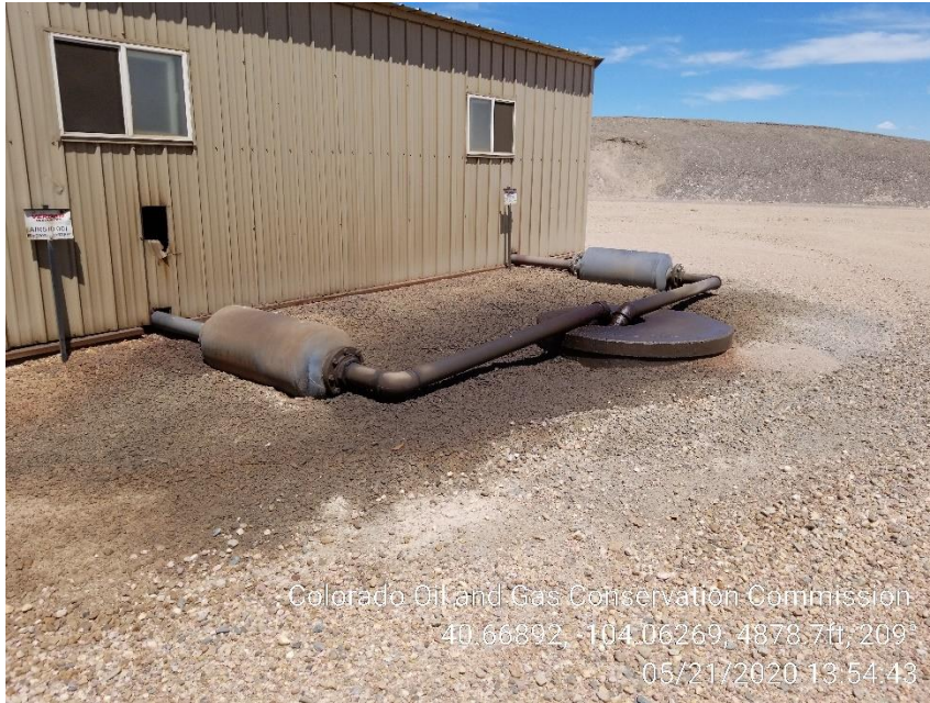
Photo 1 – Stained Soil at Engine Exhaust
