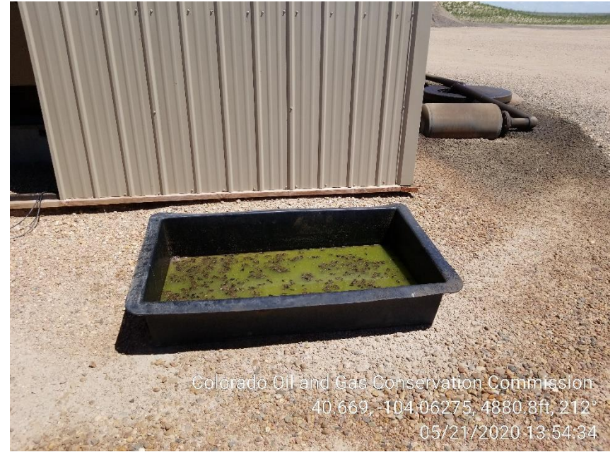
Photo 2 – Unused Secondary Containment at Pumping Units
