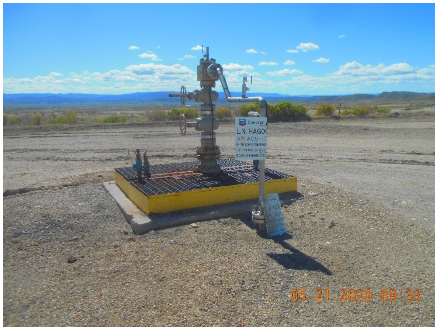
Injection wellhead
