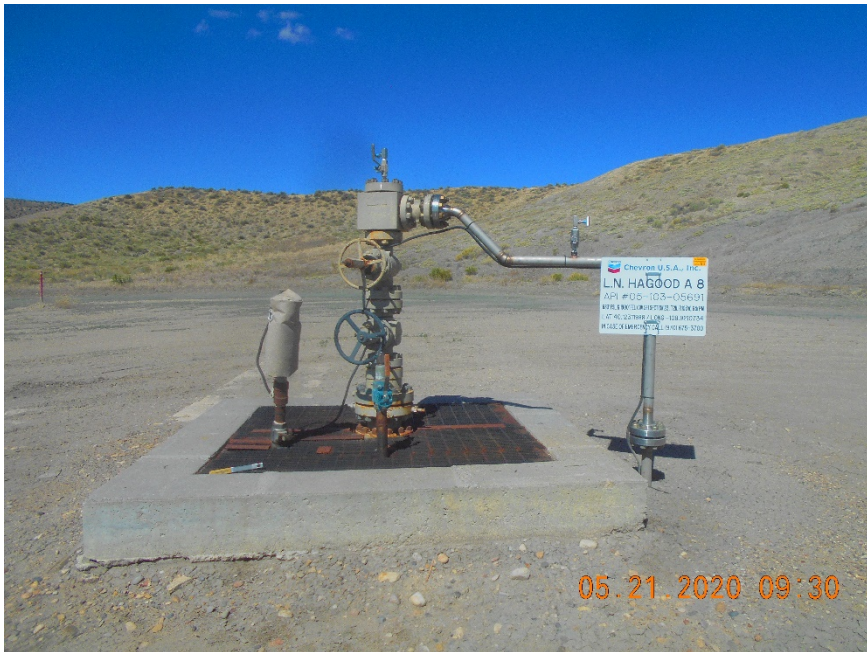
Injection wellhead
