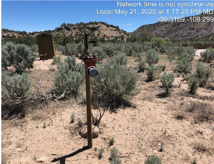
Photo #1246 Multiple flowline risers not LO/TO.
