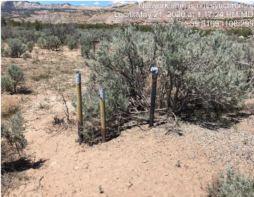
Photo #1245 Multiple flowline risers not LO/TO.
