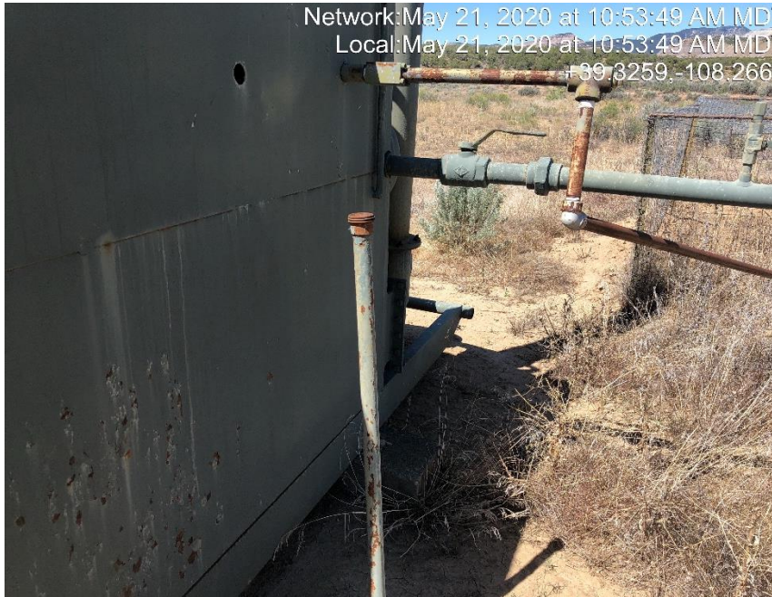
Photo #1237 Flow line risers not LO/TO.
