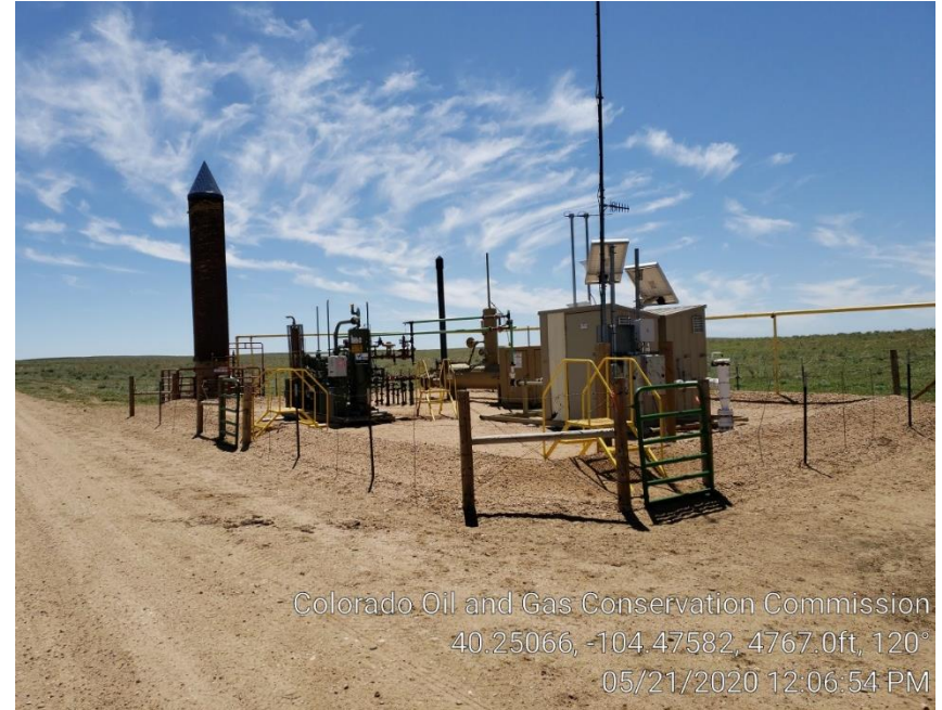
Photo #3 Separator, ECD, VRU & Meter Runs
