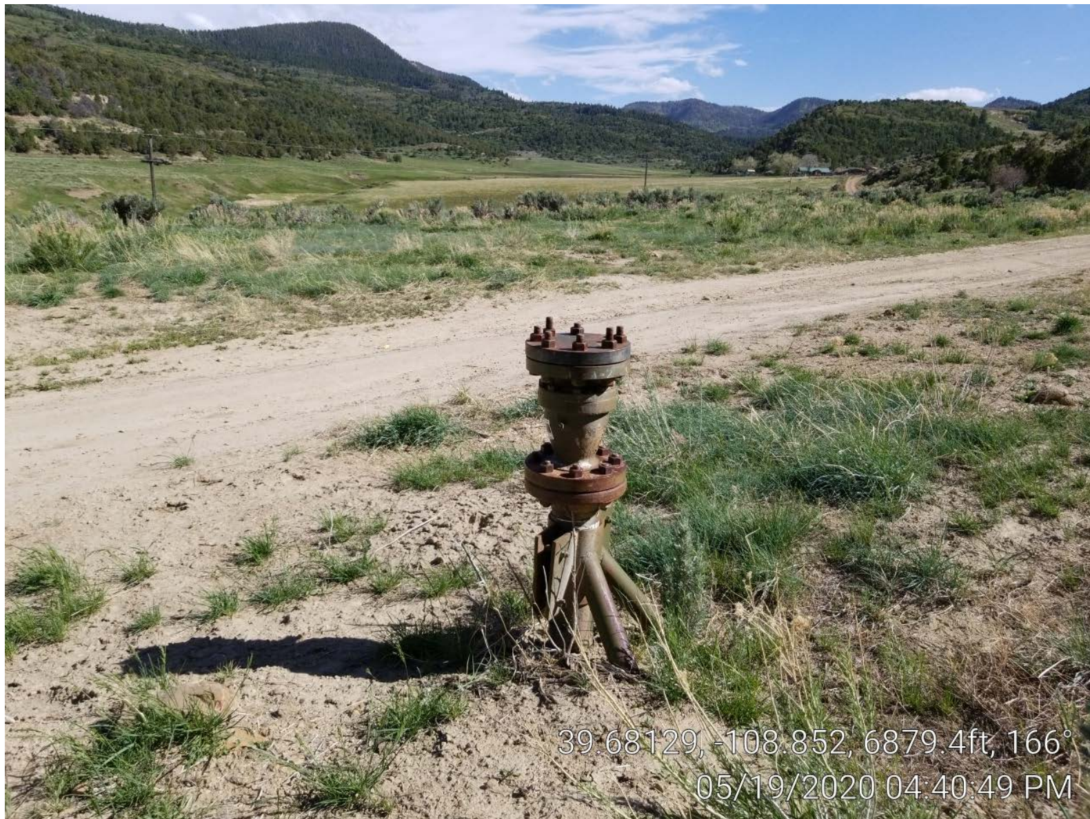
Photo 2. Location with flow line riser.
