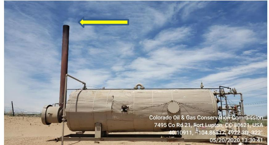
**Photo 8 Horizontal Heated Separator/ bird protector is missing**
