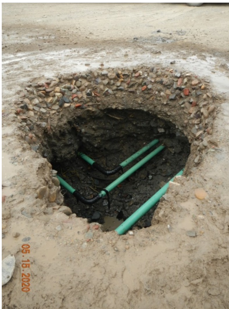
Photo#2: Excavation exposing old lines.
