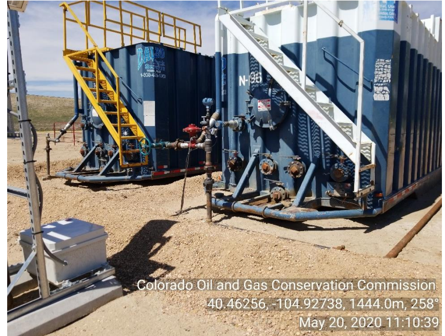
Photo 30: Tanks appear to not be grounded
