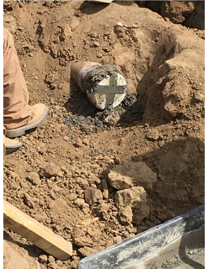
6" fiberglass final cap installed
