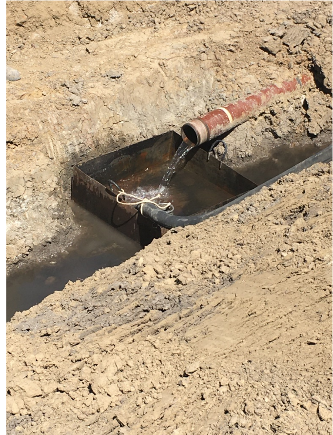
6" fiberglass being purged, 12 pigs were sent through
