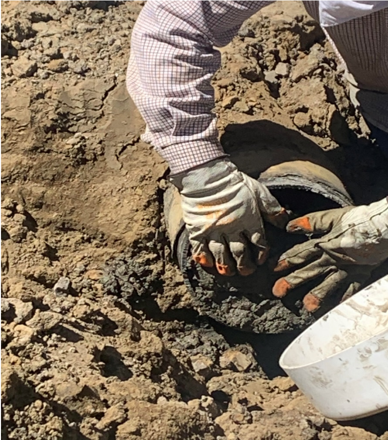
10" Carbon steel flowline dry packed with cement, foam plug was set 2' inside flowline
