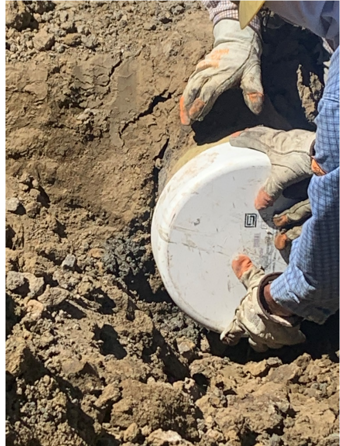
10" fiberglass final cap installed
