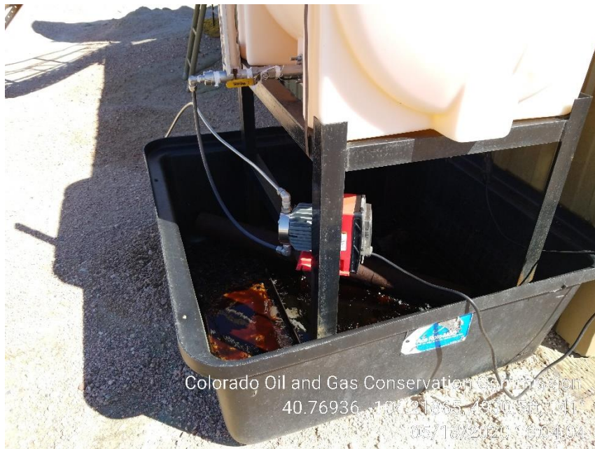
Photo 5 – No wildlife netting on Containment
