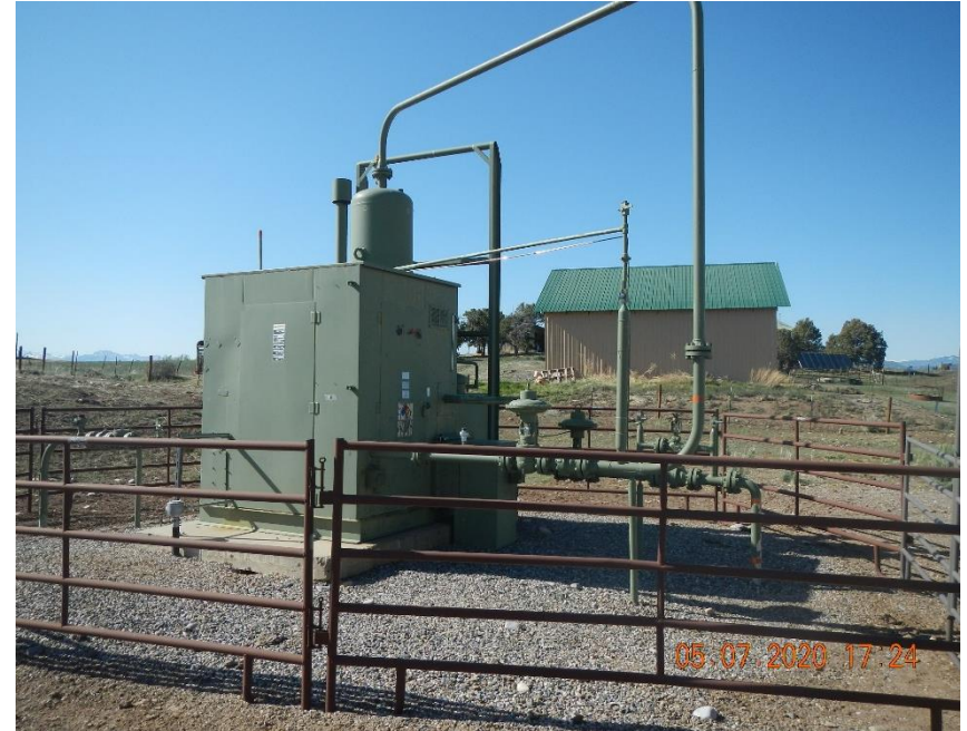
Vertical heated separator and meter run.
