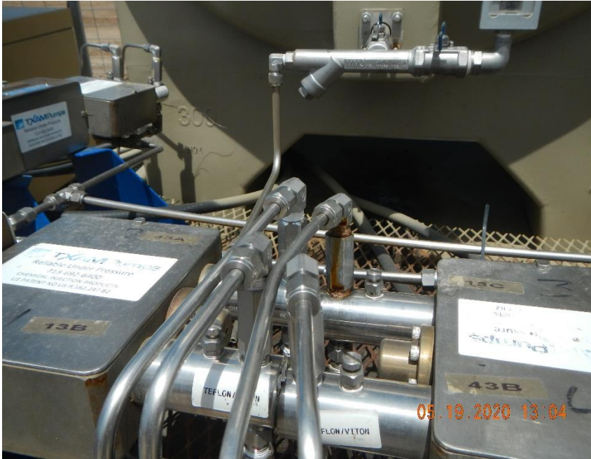
Chemical pumps on chemical containers at wells has loose fittings dripping fluid.
