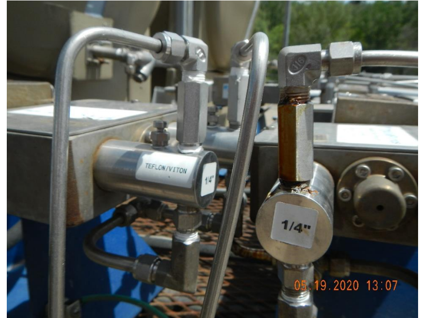
Chemical pumps on chemical containers at wells has loose fittings dripping fluid.
