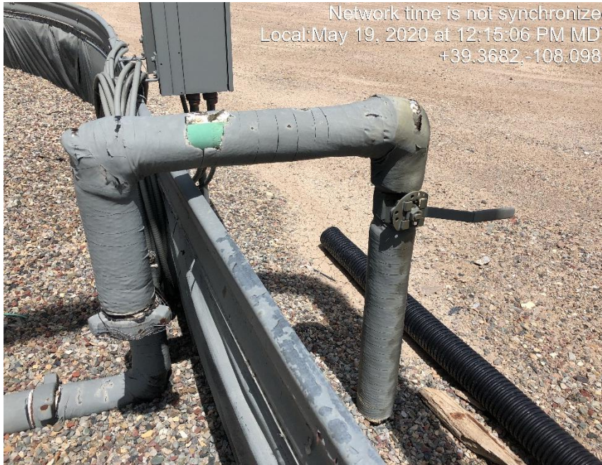
Photo #1217 Flow line riser not LO/TO.
