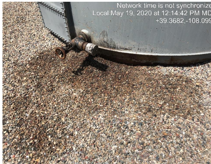
Photo #1216 Stained gravel inside tank containment.
