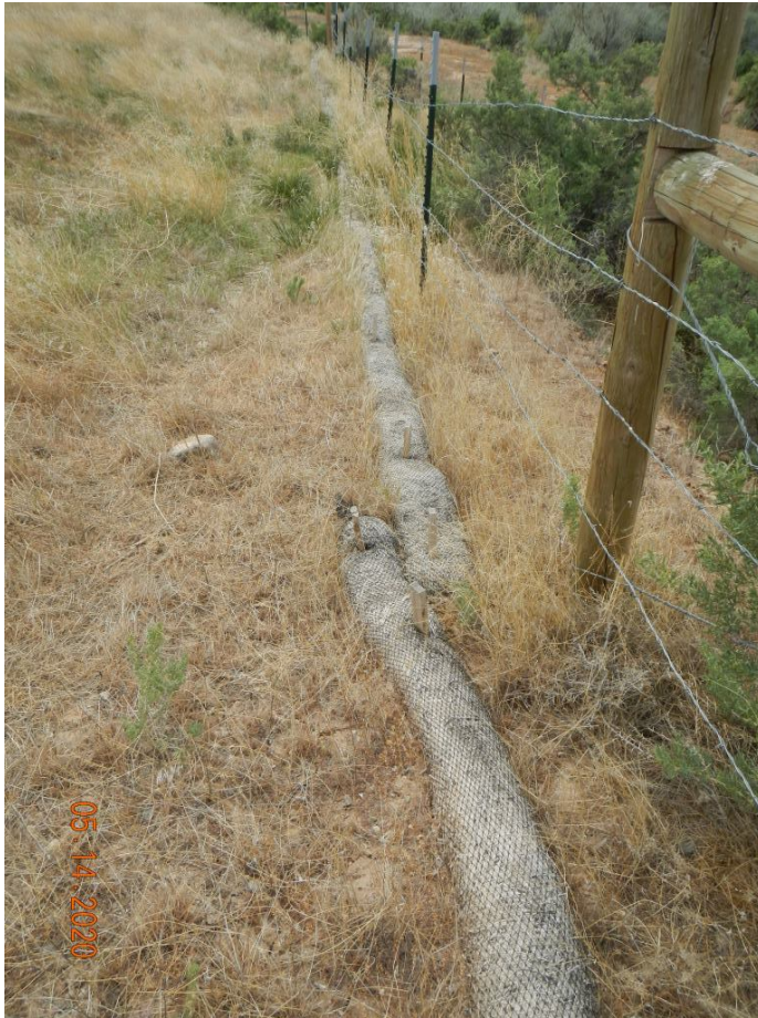
Photo#6: Wattles and subsidence repaired.
