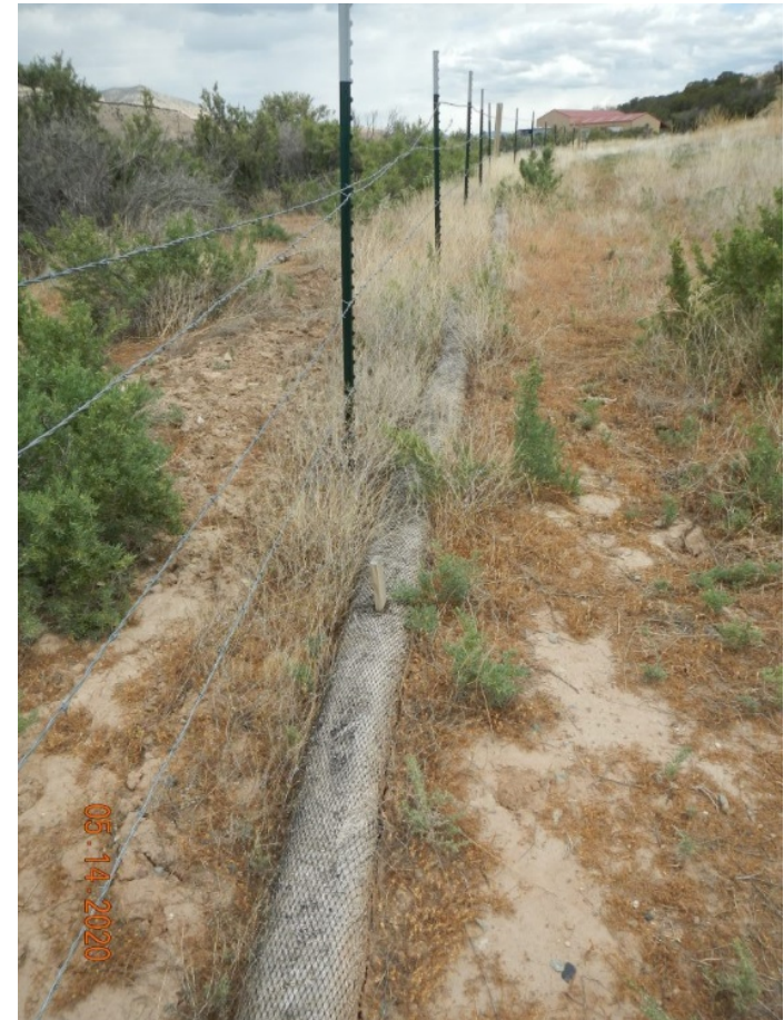
Photo#7: Wattles and subsidence repaired.
