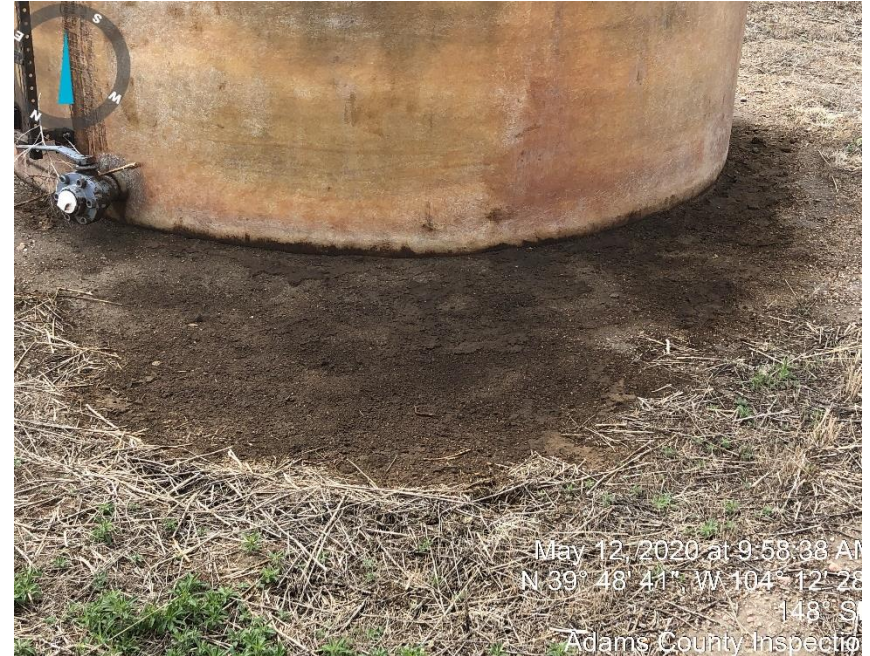
Photo #2 stained soil next to PR Water
