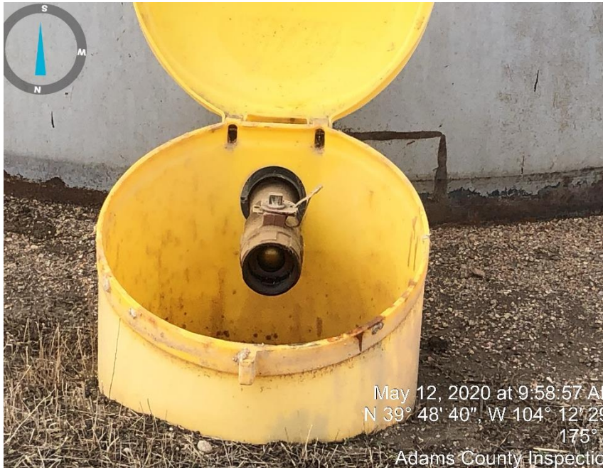
Photo #3 no bull plug in load out lines
