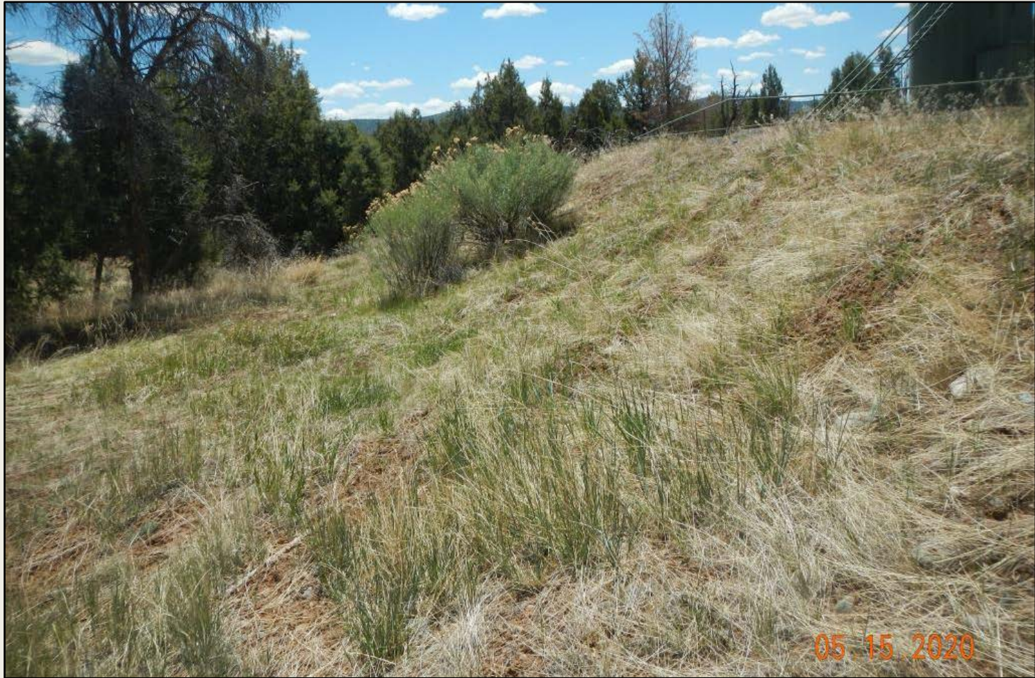
Photo 2. View of the southern fill slope from the southeastern corner facing westward. Revegetation is progressing with grasses such as western wheatgrass and smooth brome.
