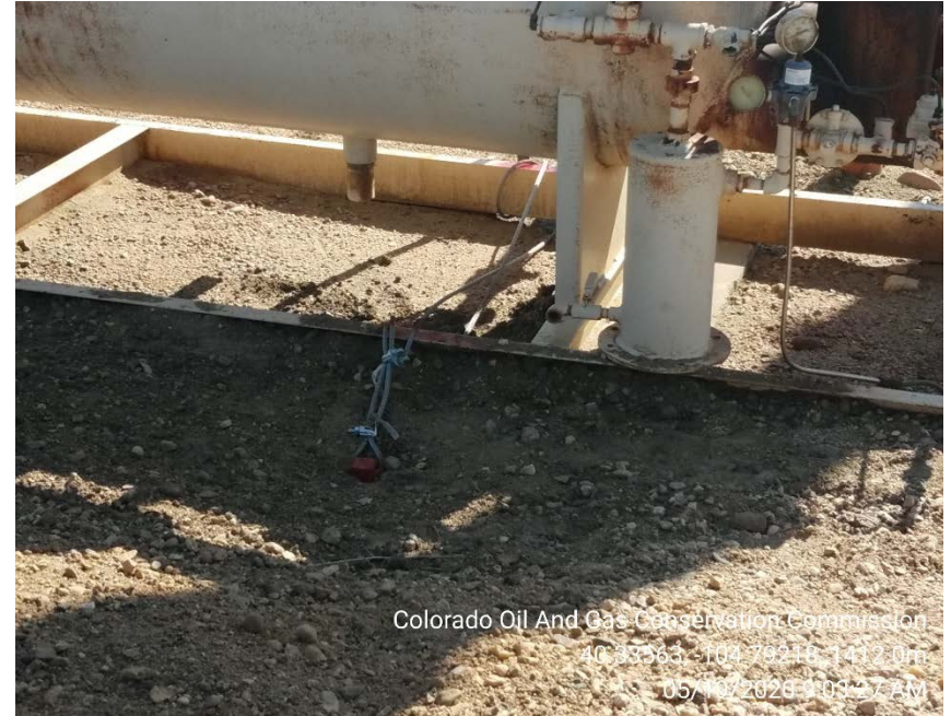
Separator anchoring
