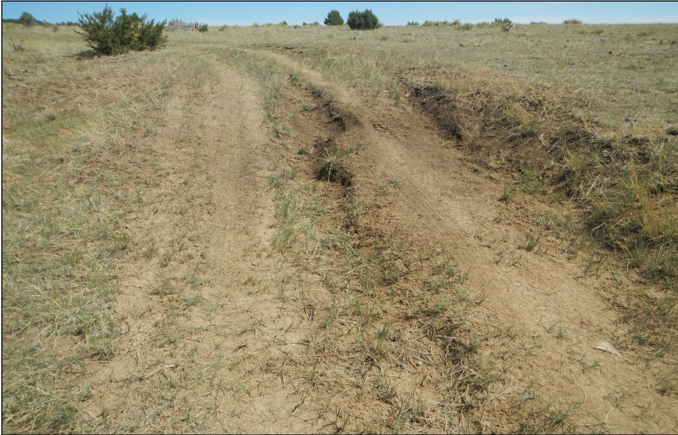
Photo 1. Facing north near the Valent Canyon location. There is an erosion channel forming along this area of the road. Lat/Long:37.34363,-104.60370.
