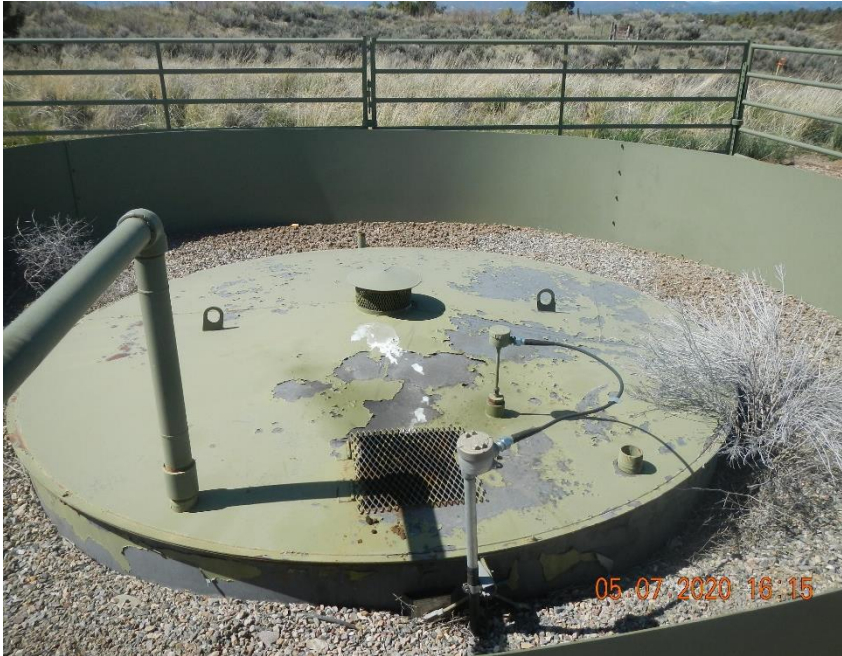
Weeds present within secondary containment ring. Paint is peeling off of PBV.
