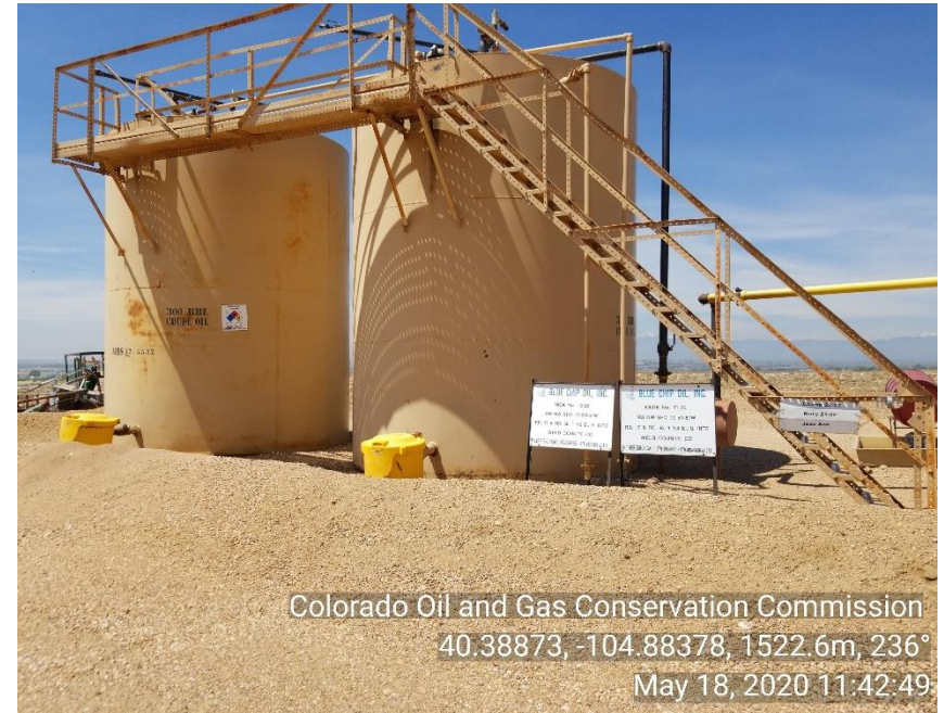
Photo 4: Tank Battery
