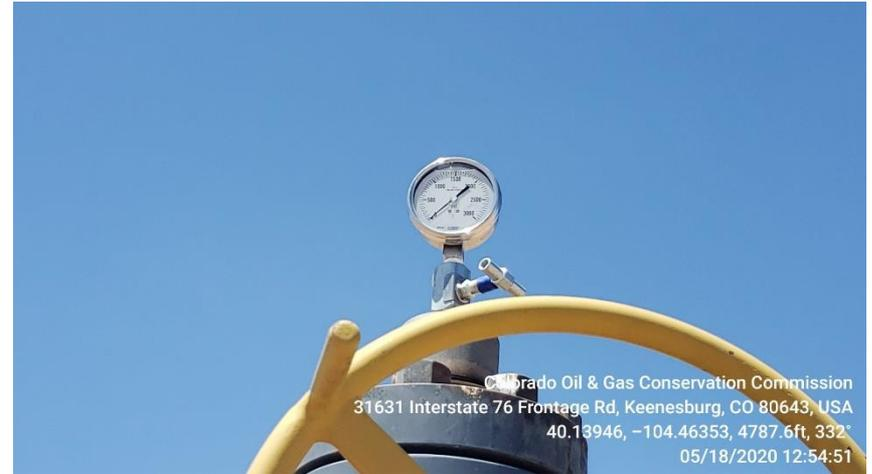
**Photo 3 Bradenhead/Casing pressure gauges reading 0 psig**
