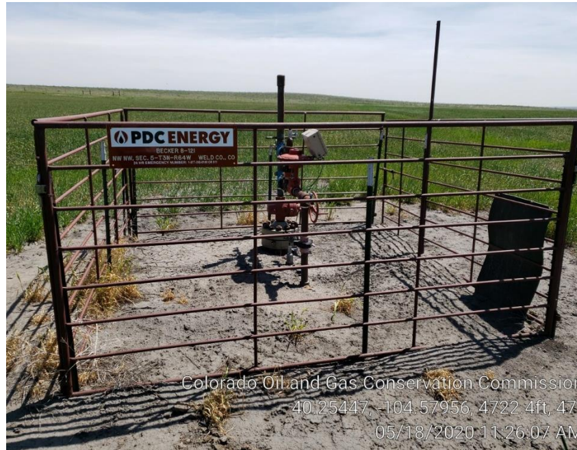
Photo #1 Well & Sign
